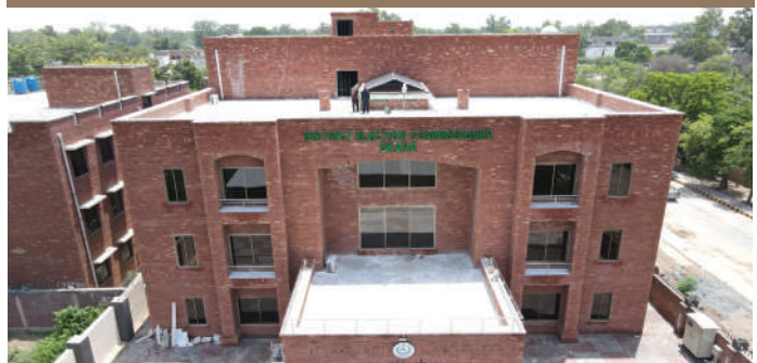
Over view of newly constructed DEC Office, Okara
